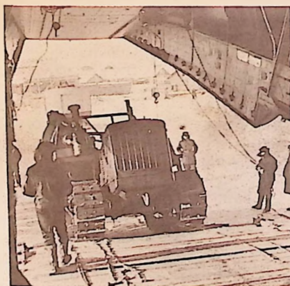
Cargo planes are used in many big construction sites in USSR. They take building machinery and heavy supplies when no other transport routes are available.
