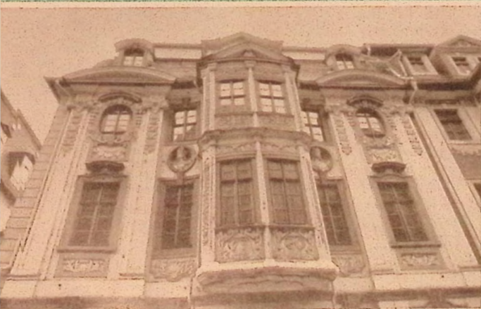
Richly decorated facade, painstakingly restored.
