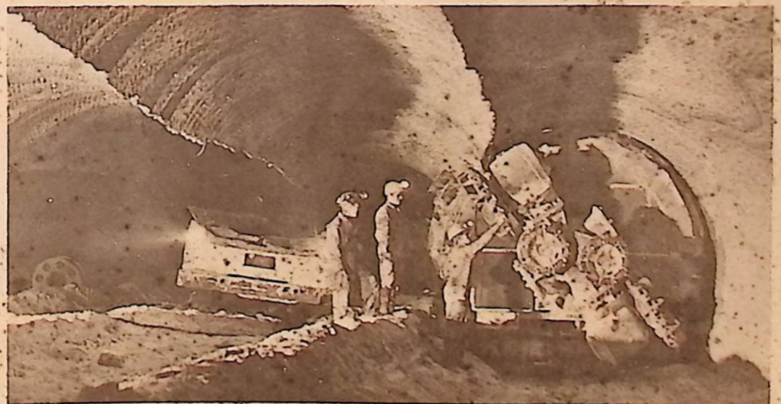
Giant Soviet-built cutter-loader at right can run by itself for hours. "Miners" (really technicians) drive on inspection tours, using special cars (one at left). Shafts are so solid that no props are required.
