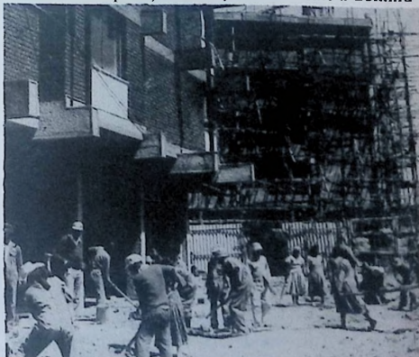
Housing construction in Addis Ababa.
