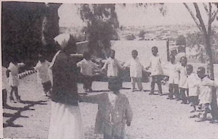
Kindergarten in Asmara.
