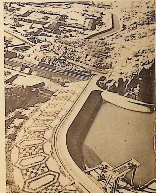
Main dam of vast Jelalabad Irrigation Complex which has for years brought prosperity to Afghan farmers.
