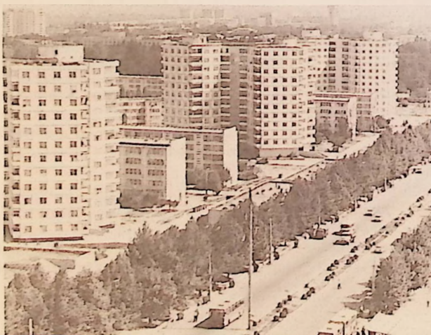
4. This is earthquake country but these new buildings are supposed to resist any shocks.
