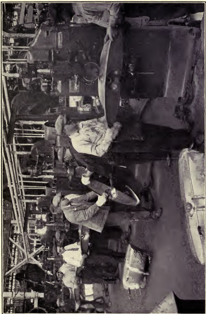
WELDING GASOLINE TANKS
