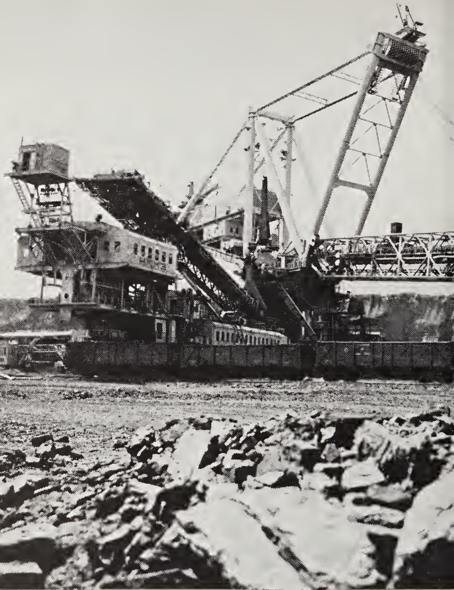
The Ekibastuz coal basin. Multi-bucket wheel excavator in the Bogatyr openpit.
