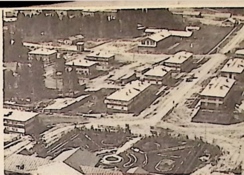
No "trailer camps" in big Siberian oil fields. Before production starts their workers get real housing.
