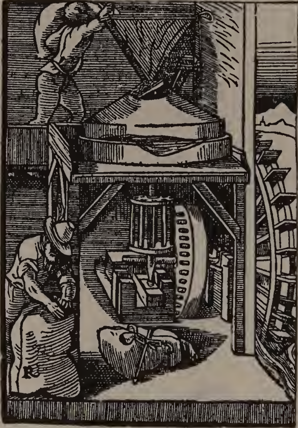
Fig. 8. Reconstruction of Vitruvius' water-mill.
