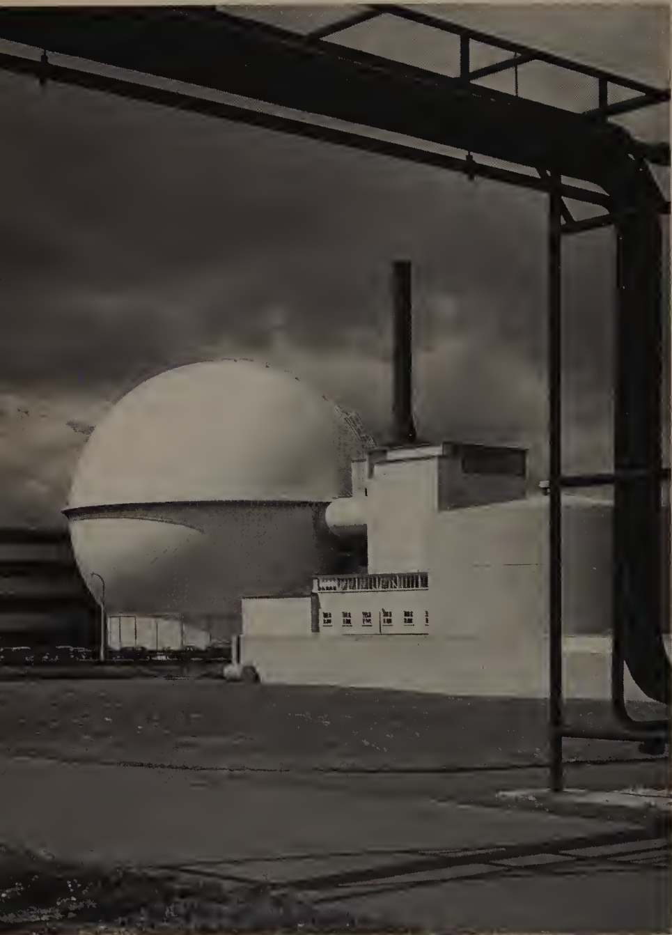
PLATE XXIX GENERAL VIEW OF THE DOUNREAY NUCLEAR POWER STATION. THE REACTOR IS INSIDE THE SPHERICAL STRUCTURE. (p. 220)
