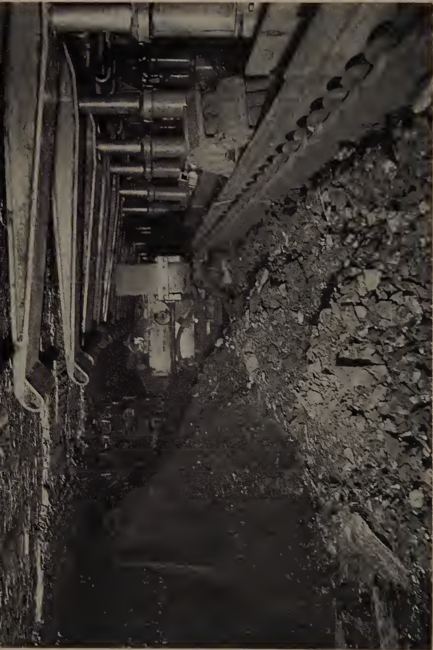
PLATE XXXIX SOVIET MACHINE FOR SINKING PIT SHAFTS, SHOWN BEFORE REMOVAL TO THE KARAGANDA COALFIELD, WHERE IT PASSED ITS TESTS. AS IT DIGS, IT LINES THE SHAFT WITH RE-INFORCED CONCRETE. (p. 270)
