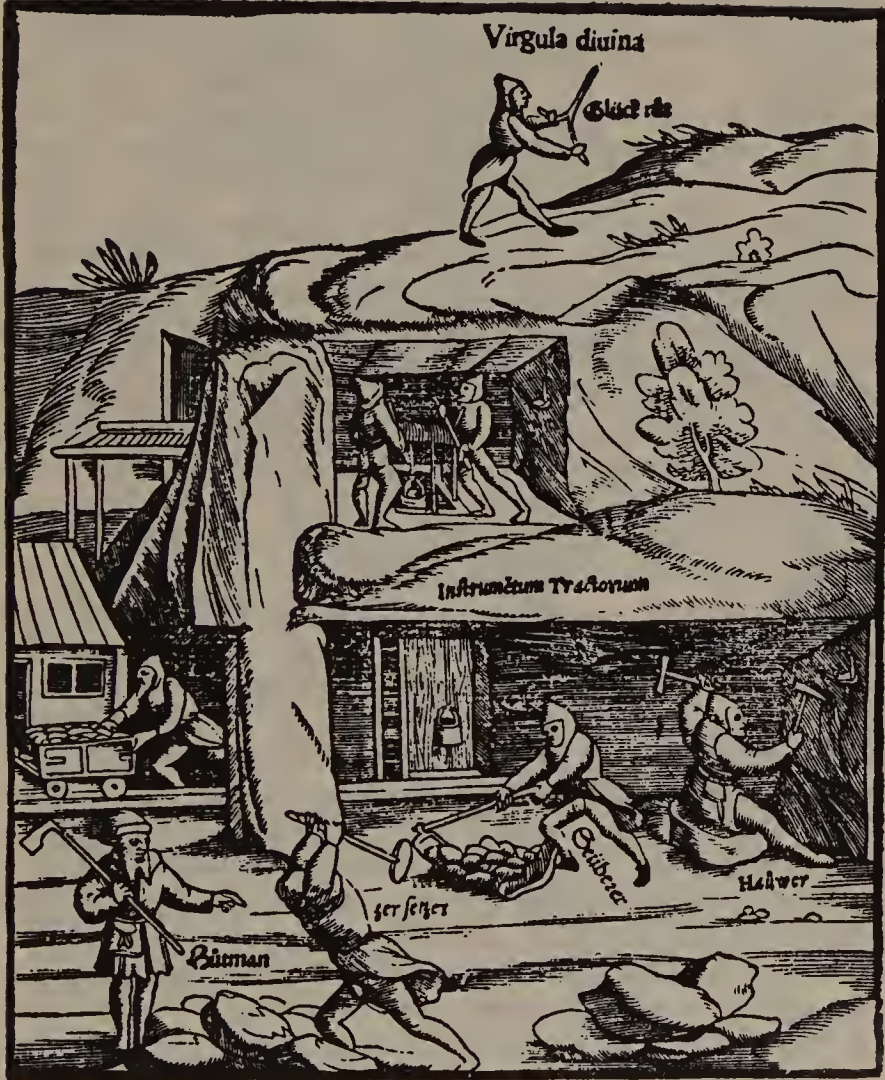
Fig. 16. A sixteenth-century minehead railway. Note also the crude winding by winch in this case.
