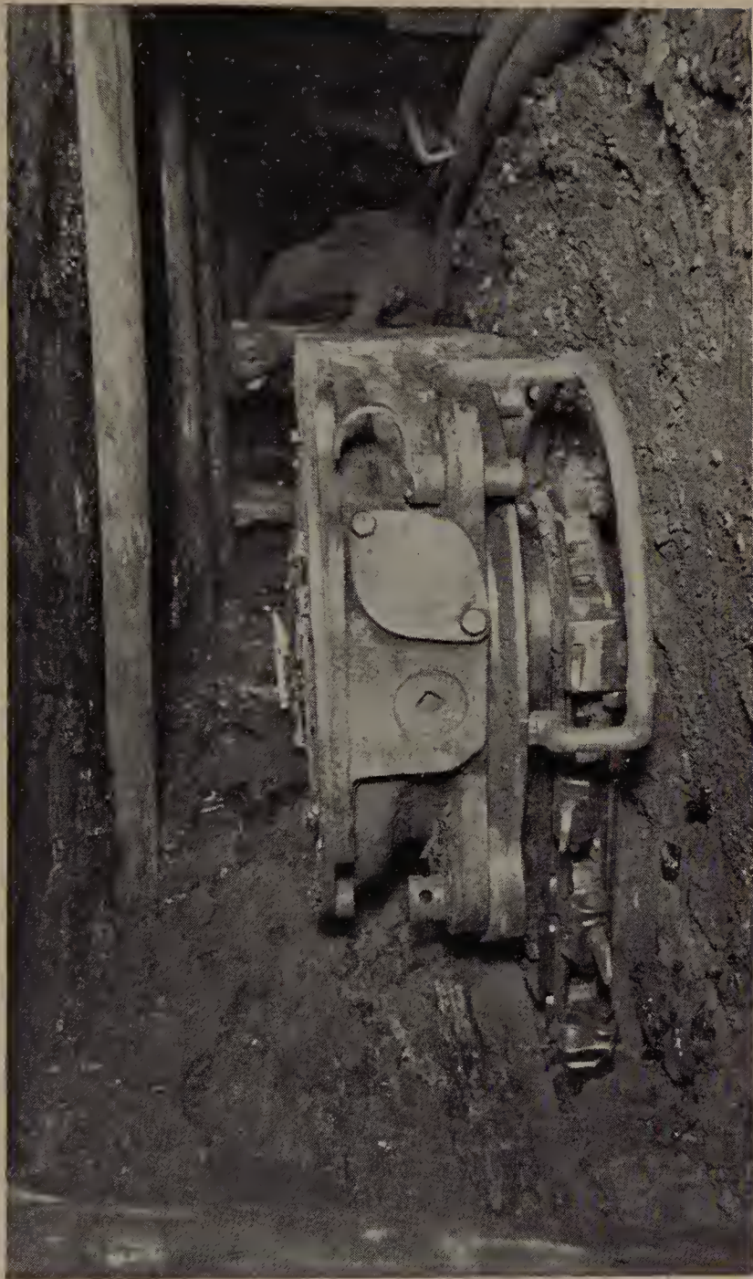
PLATE XVI A CHAIN-TYPE COAL-CUTTER. (p. 136)
