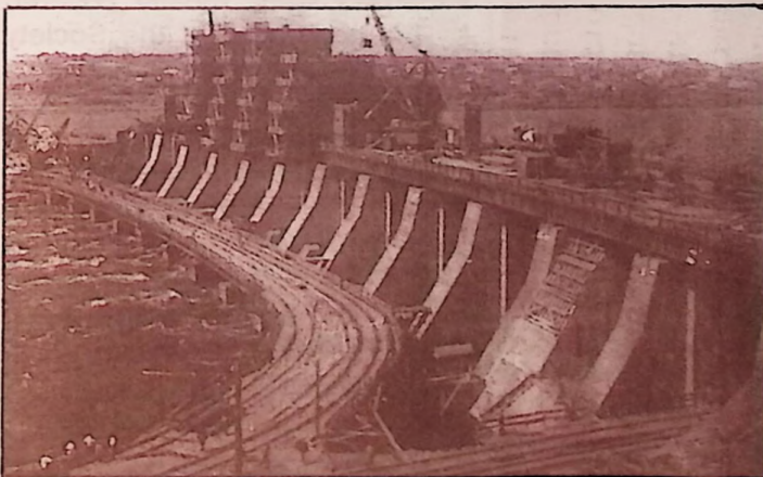
Dniepropetrovsk Dam in Soviet Ukraine, completed in 1932, supported the largest hydroelectric plant in all of Europe.
