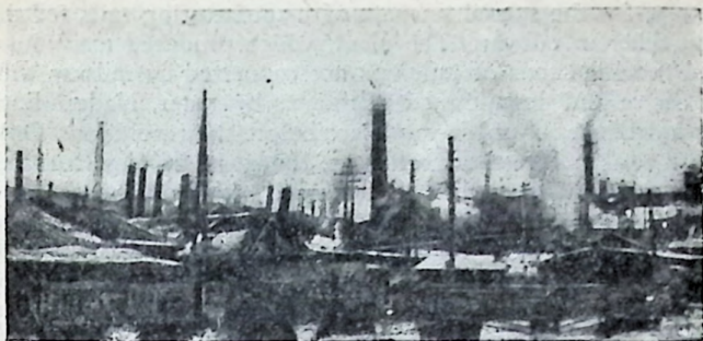
Smelting Works at Nadezhdinsk in the Urals
