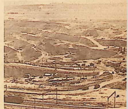
World's greatest iron-ore field now opening up, the Kursk Deposit. Steel will be made directly from ore without blast-furnaces.
