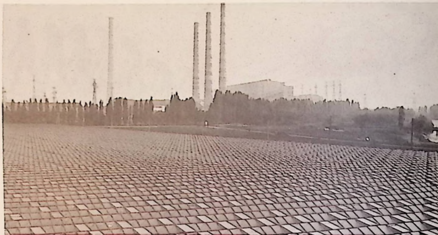
This power station at Tirasopol (Moldavia) is one of biggest coal plants in USSR. Scientists developed anti-pollution equipment to remove gases from smoke. They're converted into mineral fertilizers for enriching farmlands, 50,000 tons per year on first unit, with 11 more to come. Payoff: heat is used for greenhouses shown in foreground above.
