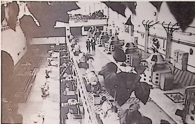
This Pumping Station handles 800,000 cubic yards per day of liquid sewage from Western and Northern sections of Moscow. Kept spotless and odorless, it works in conjunction with huge disposal plant nearby.
