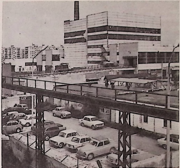
This Pumping Station handles 800,000 cubic yards per day of liquid sewage from Western and Northern sections of Moscow. Kept spotless and odorless, it works in conjunction with huge disposal plant nearby.
