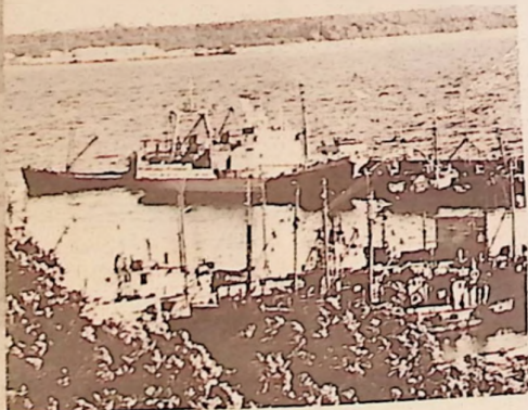
One of their larger ships, at Miidurand. Co-Op has its own ship yards and machine base for complete overhauling at lowest cost.
